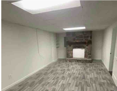
Repair FP to working order
