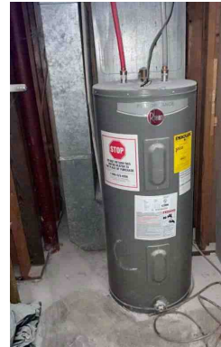
Water pan to be installed
