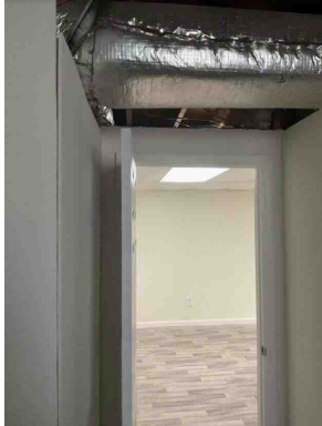
Secure wiring/pipes;finish laundry
