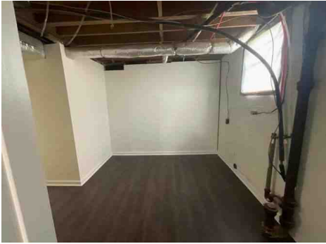
Secure wiring/pipes;finish laundry
