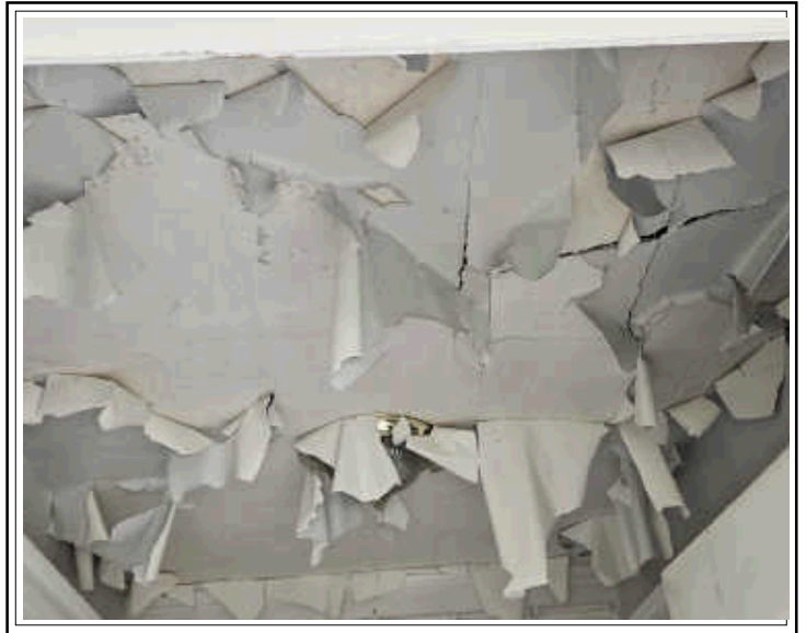
Scrape and paint ceiling Unit 1
