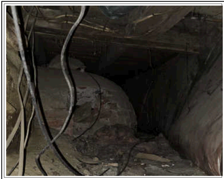
Crawl space area
