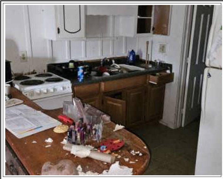
Second view kitchen Unit 1S
