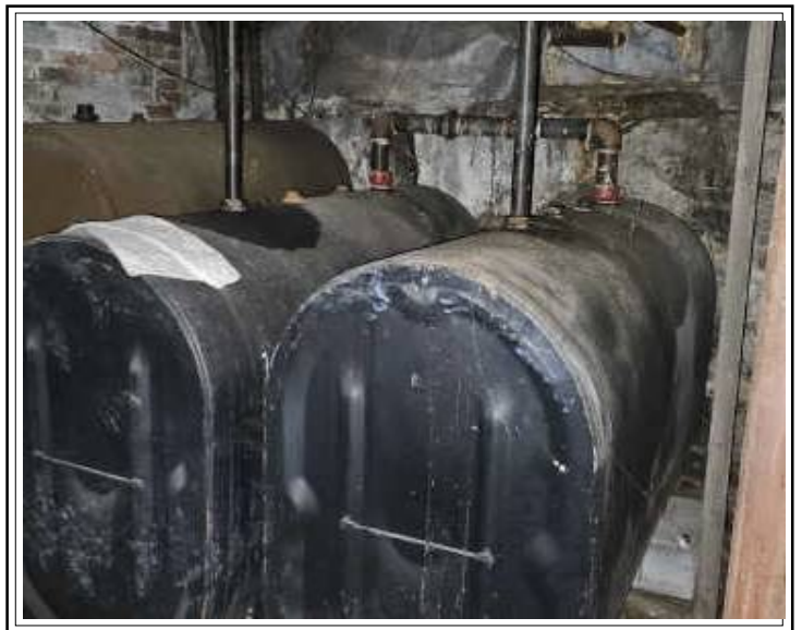
Location of oil tank basement
