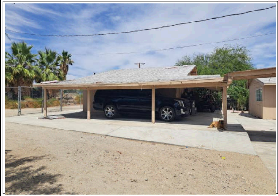
Detached 1 car carport & the unpermitted 2 car garage conversion
