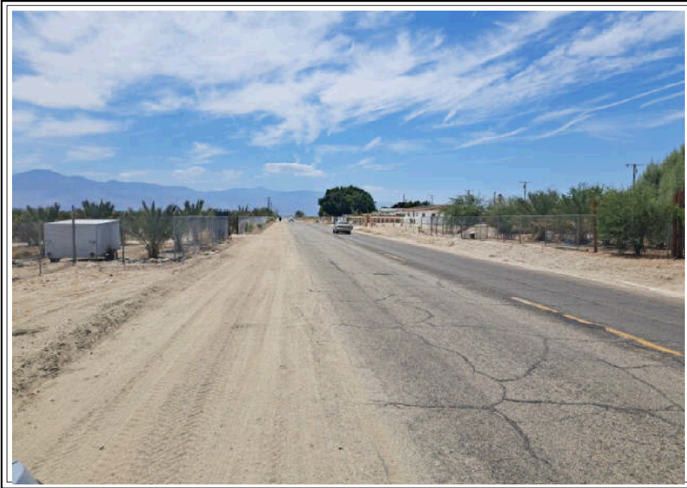
Another street scene facing west
