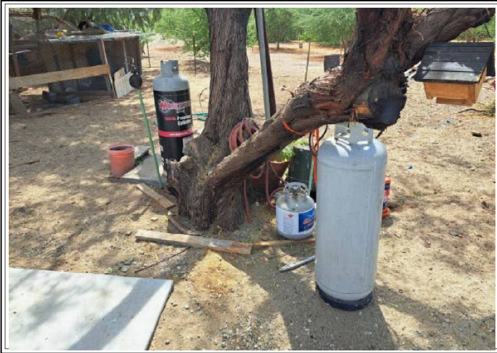
Free standing portable propane tanks Need Straps - Health & Safety issue
