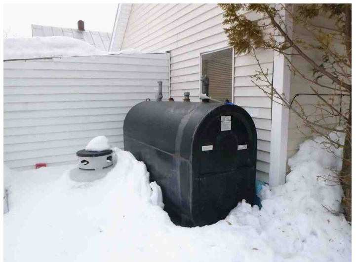
Oil Tank Outside-no sign of leakage or odor
