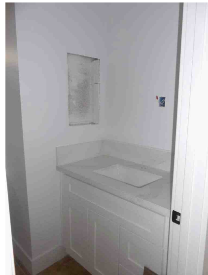
Bathroom #2 Second Floor
