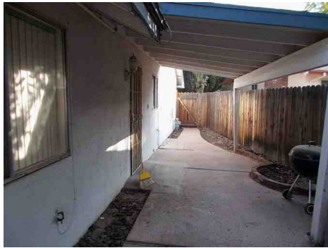
Left side of exterior
