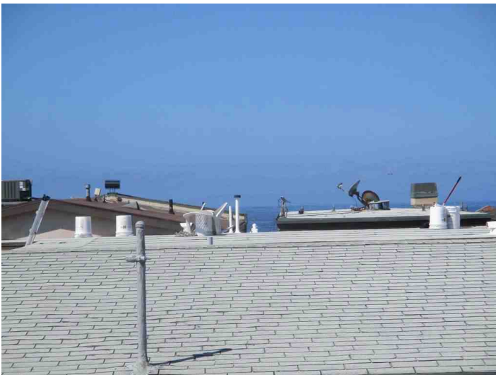
Peak Ocean View from Rooftop Deck
