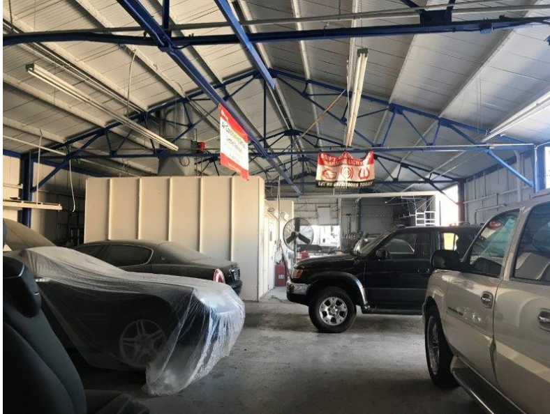
Typical View of Subject Warehouse Area
