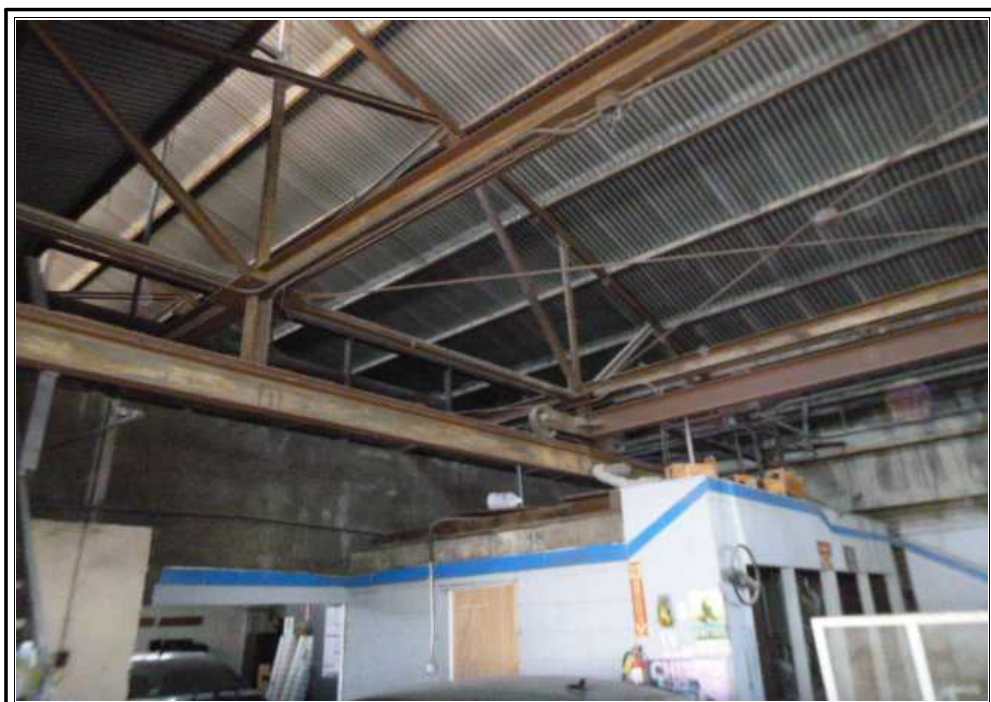
Larger Front Building Crane
