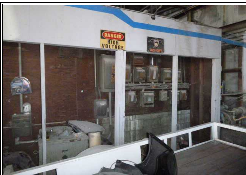
Larger Front Building Interior
