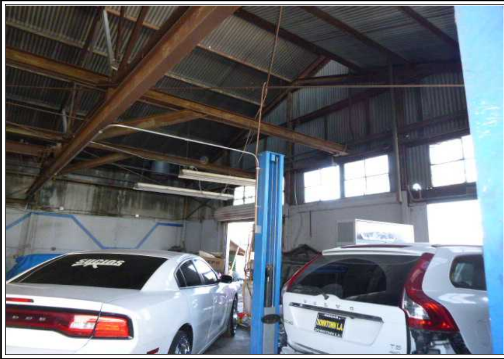
Larger Front Building Interior
