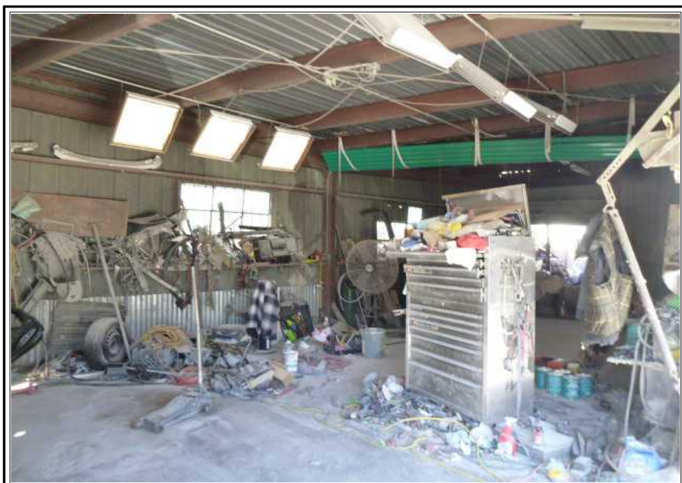
Rear Building Interior
