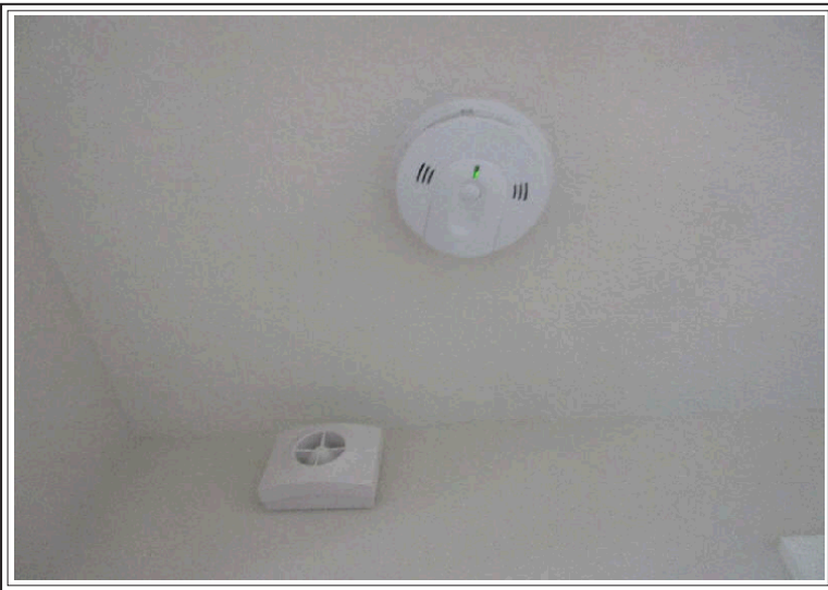
Smoke alarm/CO detector
