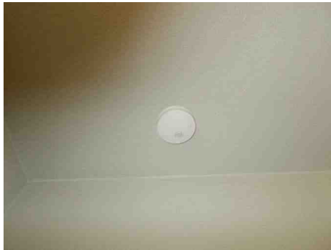
Subject Smoke Alarm
